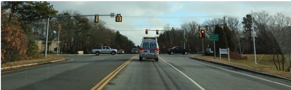
Fig. 7 – Route 151 at Sandwich Road (Facing East)
