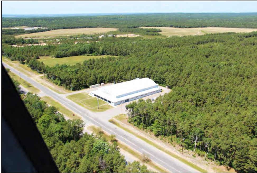
Figure 4.2: Gym Expansion – Existing Conditions (looking NW)
