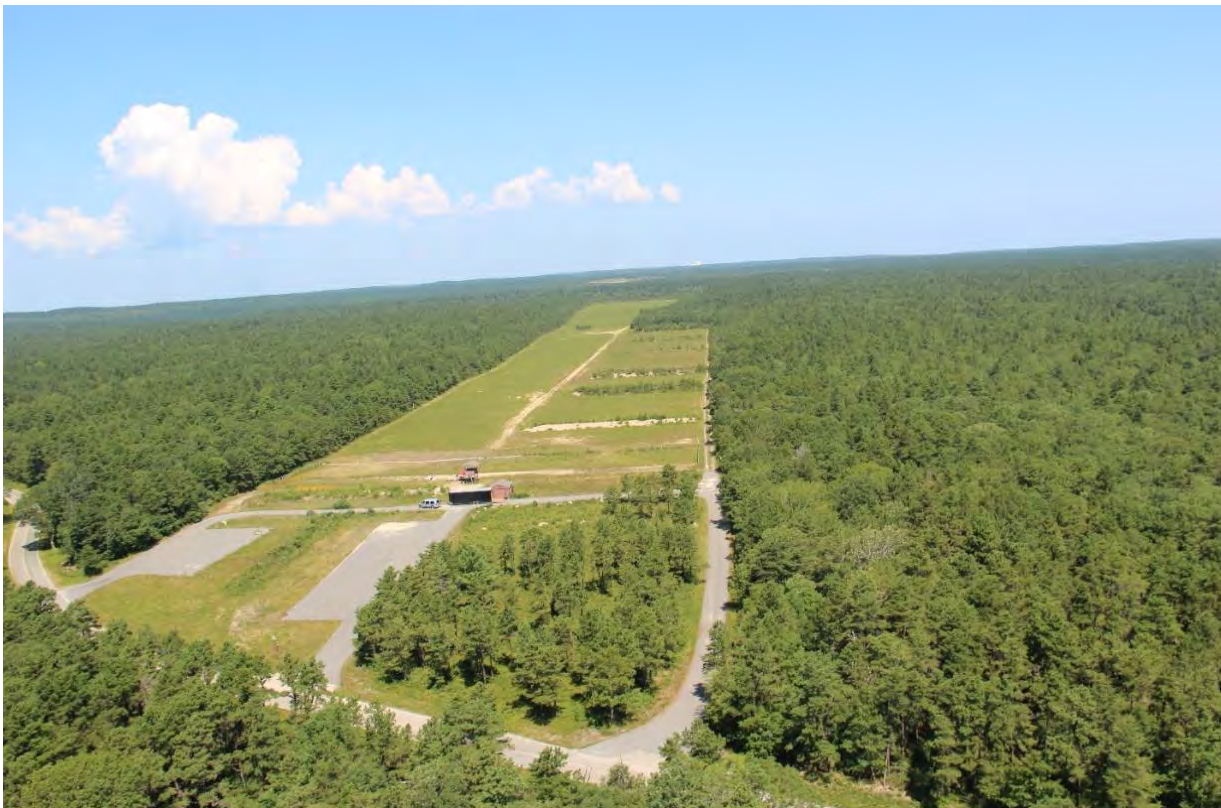
Figure 3.1: Existing KD Range looking North
