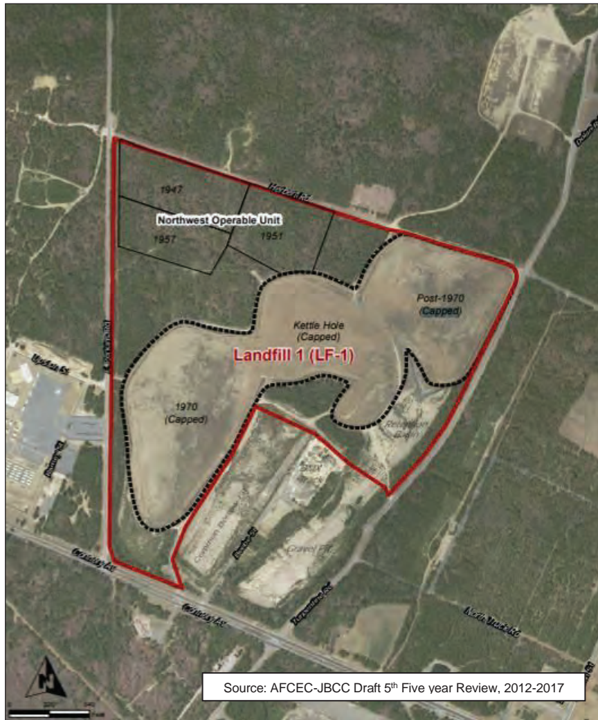
Figure 4.8: Capped Landfill Solar Array
