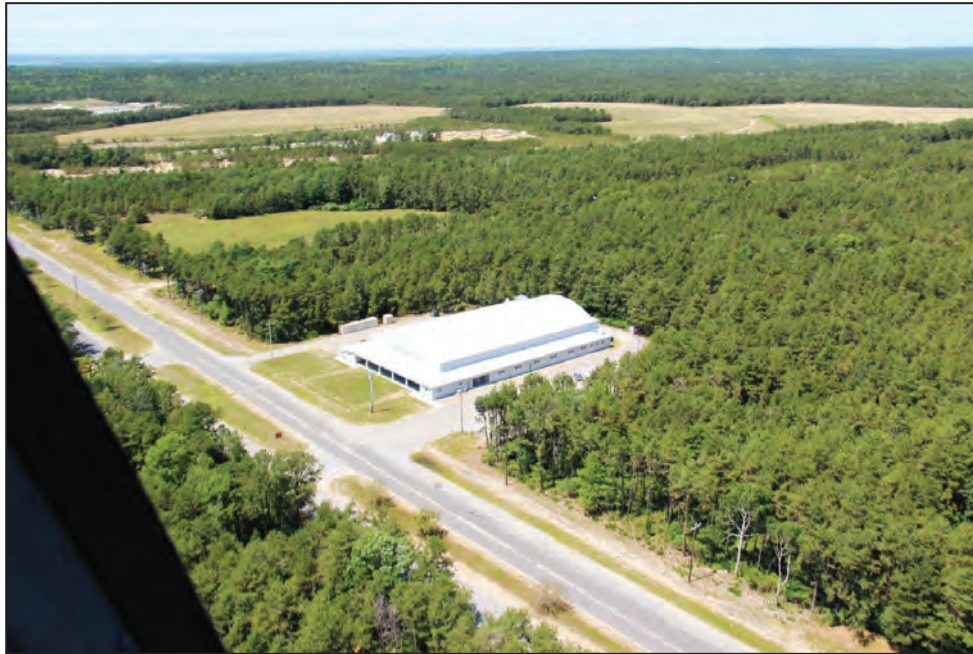
Figure 4.2: Gym Expansion – Existing Conditions (looking NW)
