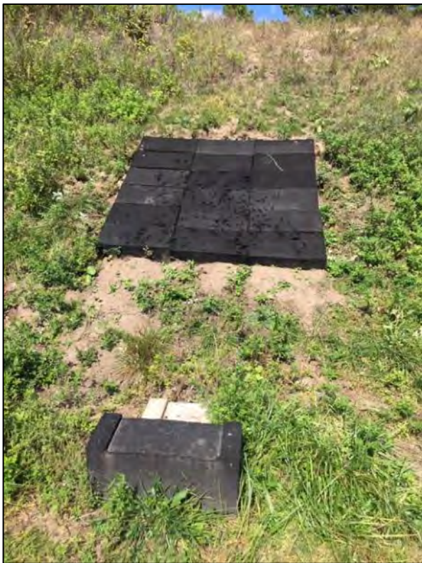
Photograph 2-1 and 2-2 Dura-Bloc™ installed on India Range as an alternative bullet pocket management.
